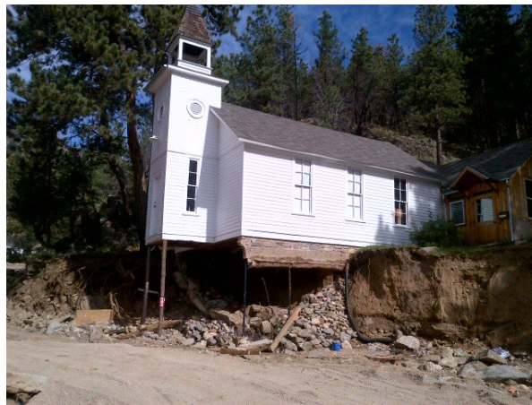
Figure 3. Structures 45+ years may require consultation with SHPO or THPO. FEMA photo.
