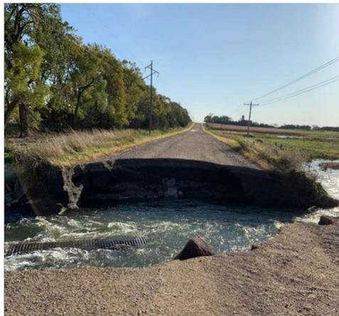
**Figure 2. Work in water due to a road collapse may require US Army Corps of Engineers NWP or 401 or 404 permit depending on the method of repair. FEMA photo.**
