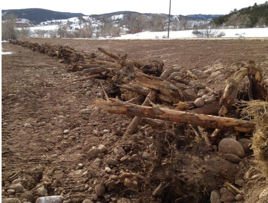
Figure 4-7: Bioengineering Using Engineered Woody Debris
