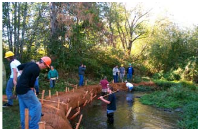
Construction of the brush mattress underway.
