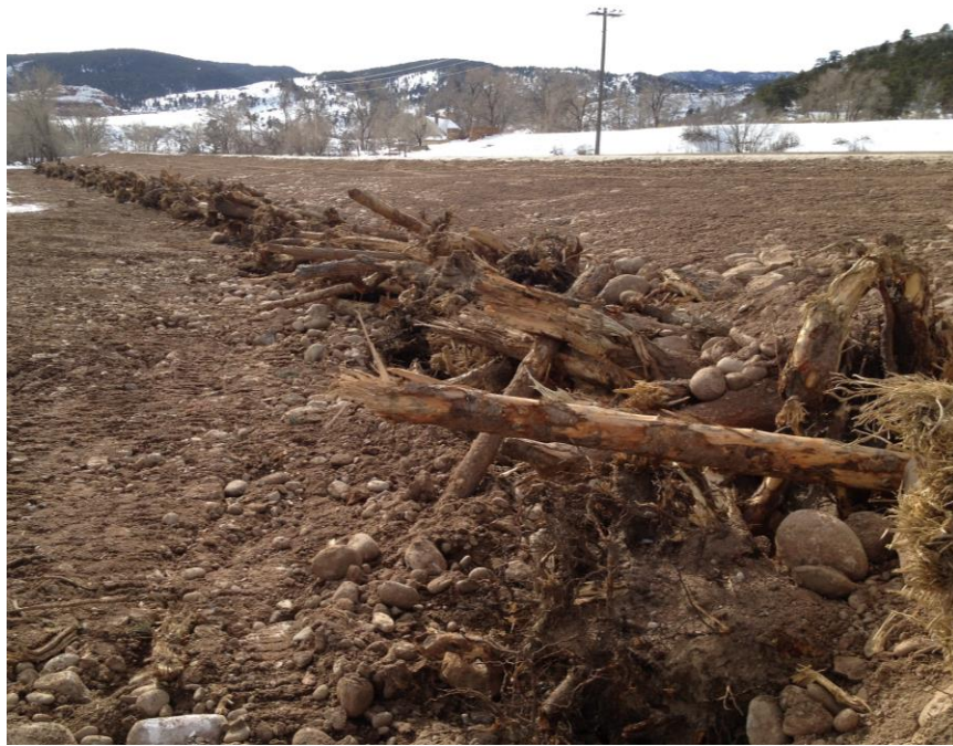
Figure 4-6: Bioengineering Using Engineered Woody Debris
