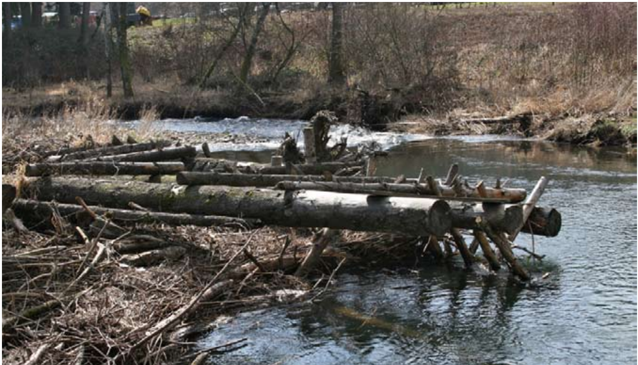
The porous design of the debris catcher allows fish to swim through the structure unimpeded.
