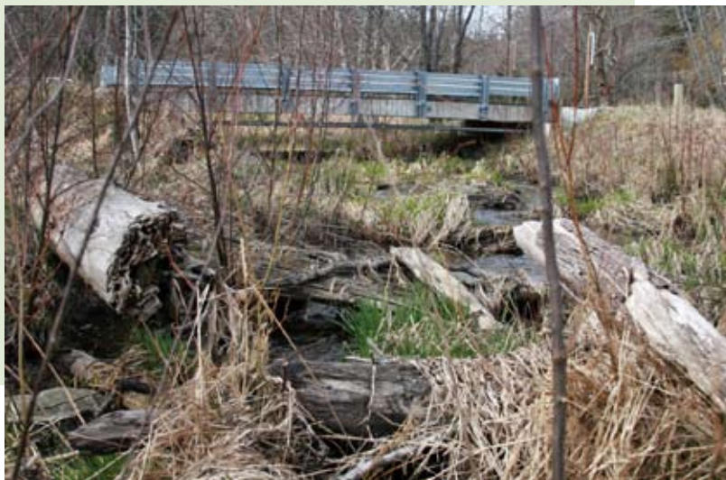
Wood positioned downstream of the bridge slows water flow and provides habitat for fish and other wildlife.
