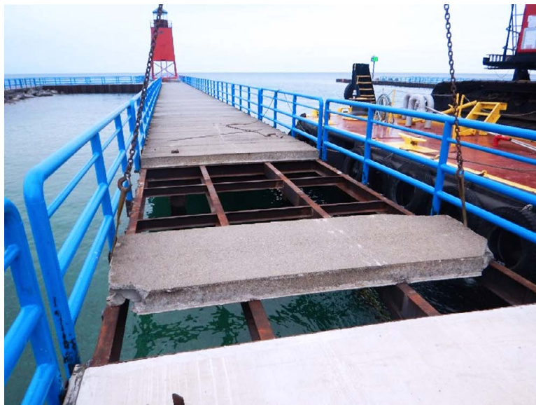
Figure 5.5.3. Improve pier performance during future storms by replacing storm-damaged pre-cast concrete pier deck panels with reinforced cast-in-place concrete (Source: U.S. Army Corps of Engineers, No Date).
