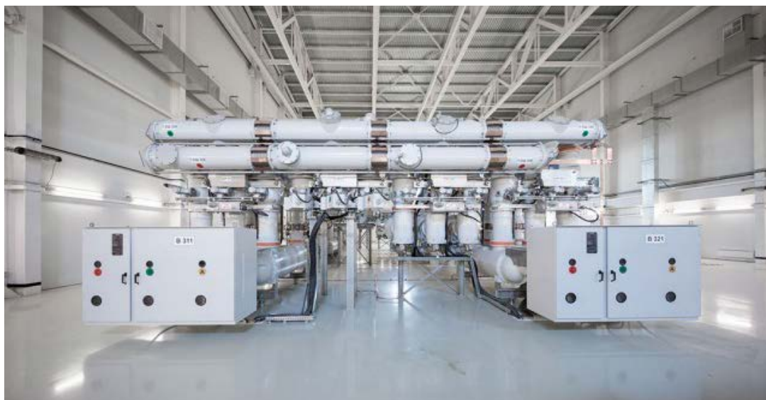
Figure 4.3.11. Indoor gas-insulated switchgears can be used in environments where water can penetrate the control house. (Source: Siemens Energy, 2021)
