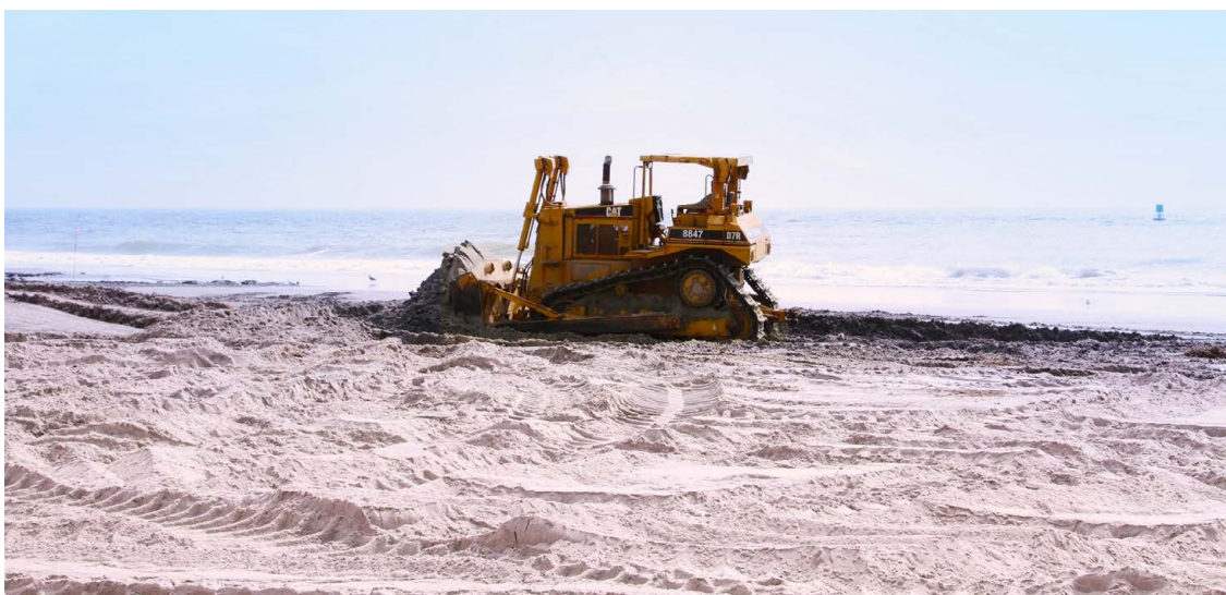
Figure 5.4.7. Beach nourishment replaces sand lost through longshore drift or erosion and increases resilience. (Source: USACE, 2020).
