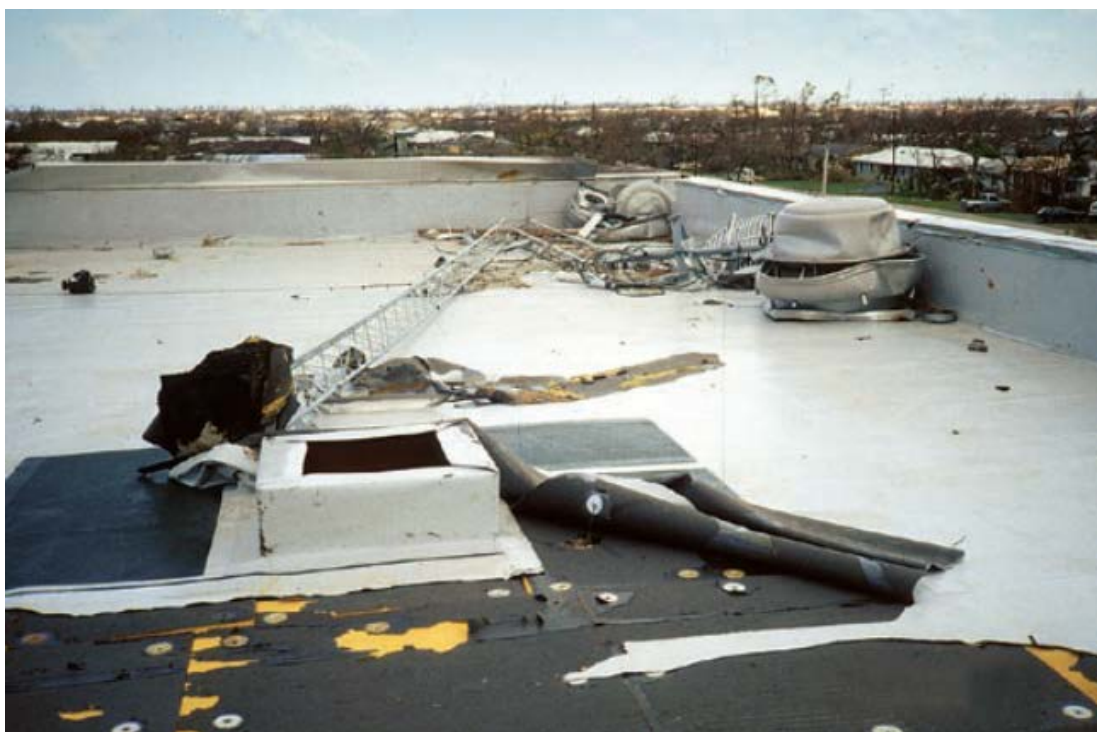
Figure 4.4.1. The collapse of a tower with antennas can damage the roof membrane, causing it to peel.
