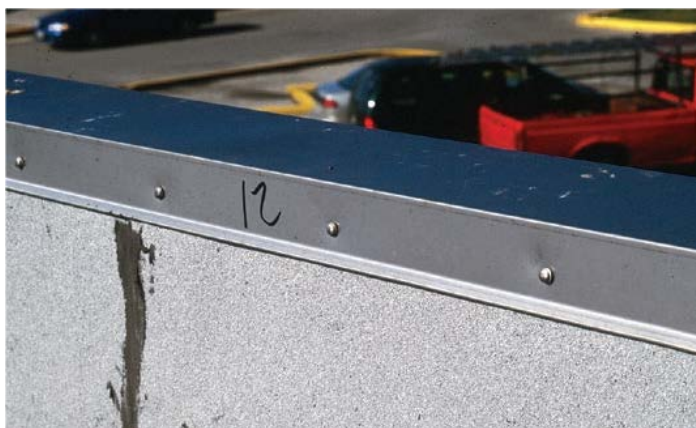
Figure 3.3.2.3. Both vertical faces of coping were attached with exposed fasteners ( \frac{1}{4} -inch diameter stainless steel fasteners spaced 12" on center) instead of concealed cleats following Typhoon Paka (1997) in Guam to prevent the flashing from tearing in future storms.
