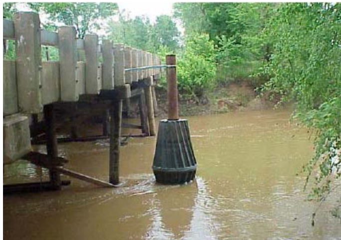
Figure 1.4.20. Pile-mounted debris sweepers can effectively direct debris away from bridge piers (FHWA, 2005).
