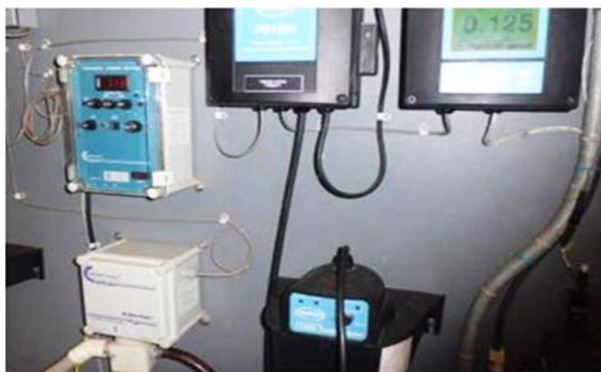
Figure 4.1.6. Elevating instrumentation can protect it from flood damage. (Source: U.S. Environmental Protection Agency [EPA], 2014)
