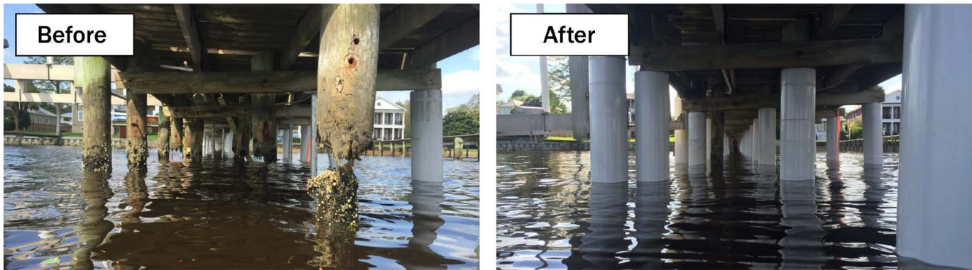
Figure 5.5.2. Fit aging piles with jacket encasements to strengthen and protect them (Source: Shoreline Plastics, No Date).
