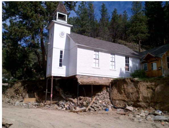
Figure 3. Structures 45+ years may require consultation with SHPO or THPO. FEMA photo.
